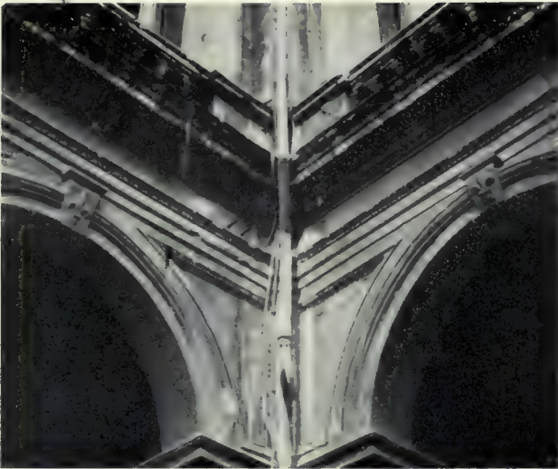
29. - Palazzo Borghese. Court, detail of keystones in east corner.
